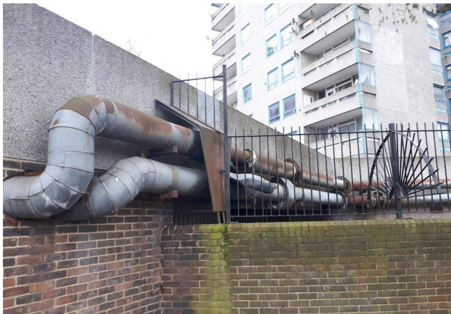
Figure 25: Example of above-ground DH pipework, mounted on side of Parkview Estate podium walkway
