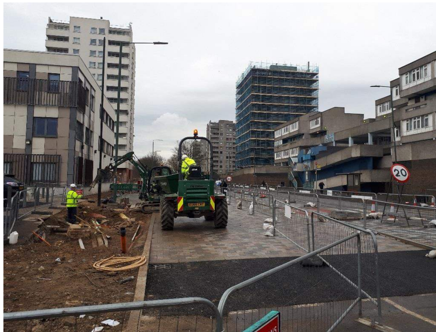
Figure 24: Ongoing enabling works within Yarnton Way (east of A2041 roundabout)
