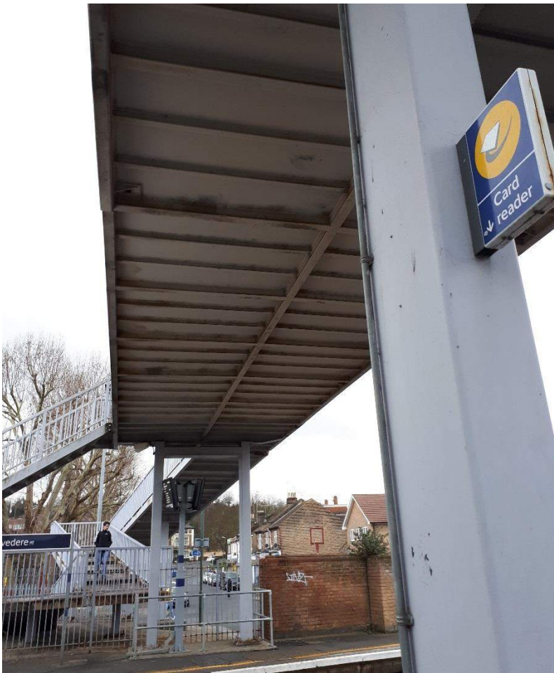
Figure 27: Pedestrian footbridge at Belvedere station
